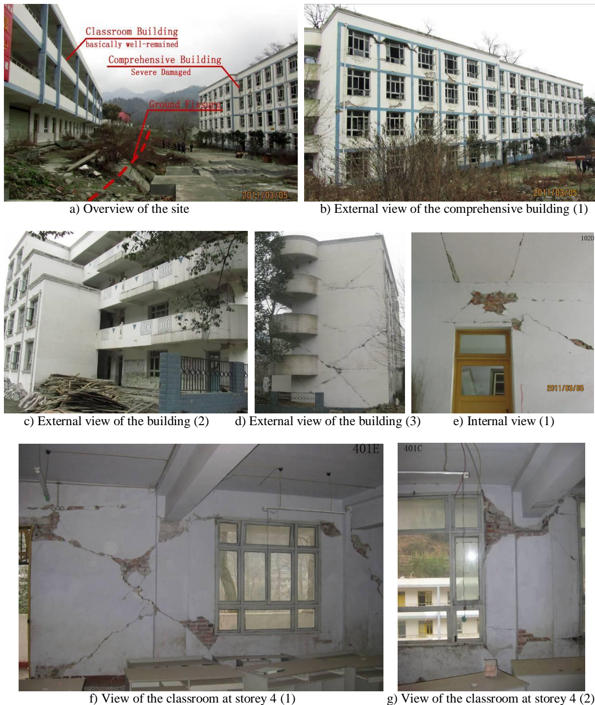
Fig.1 Overview of White Deer Middle school earthquake damaged site and typical damage appearances of the comprehensive building
