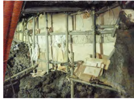
(2) Mortar-bag bulkhead
