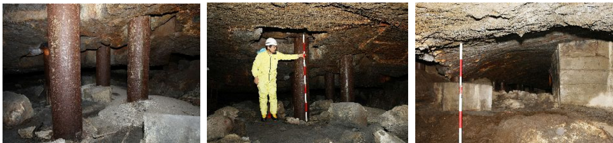
Photo 3. Steel-pipe piles for the city hall driven through lava tubes
