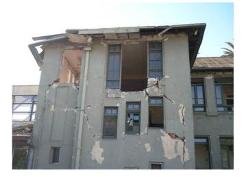
Figure 1.1. Crack pattern in infills wall with opening.
