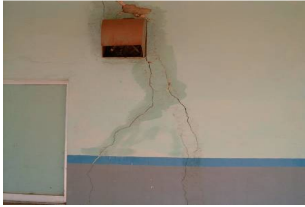
Figure 10. Cracks in the walls
