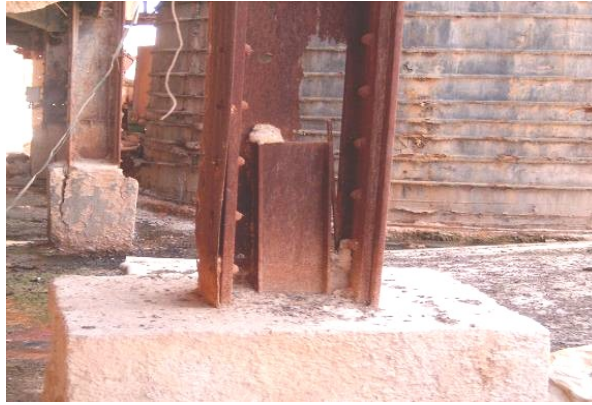
Figure 3. Corrosion of columns
