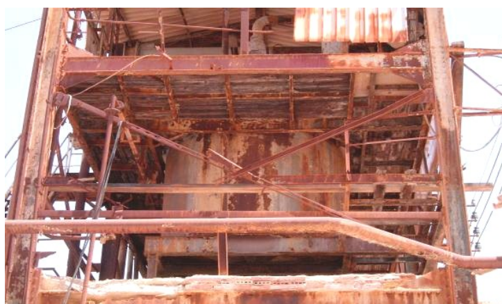
Figure 2. Damage in the bracing system
