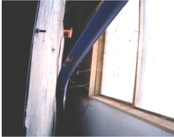
Figure 7. Instability of the bracing system
