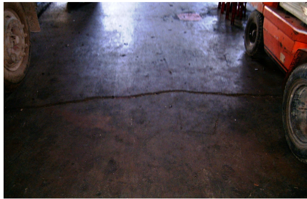
Figure 11. Cracks in the pavements
