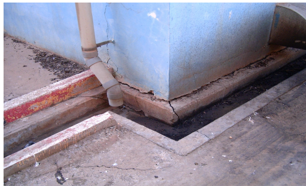
Figure 8. Hole in the joints
