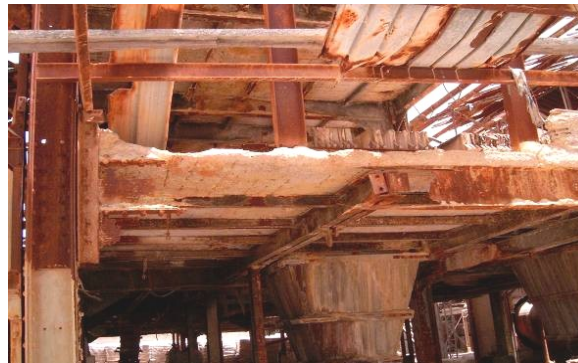
Figure 5. Damage in beams and floors
