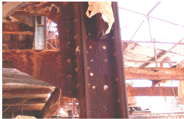
Figure 4. Damage in the assembly system
