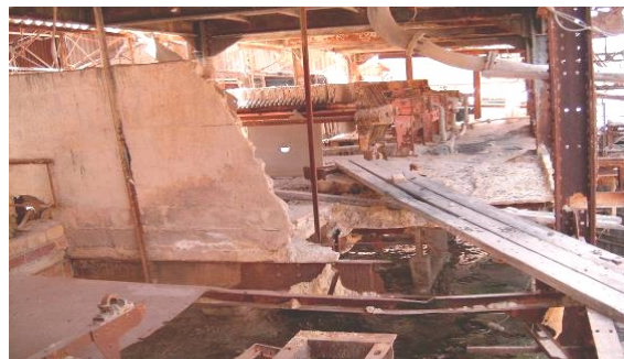
Figure 6. Collapse of a floor
