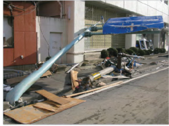
Figure 17. Failed sign structure
