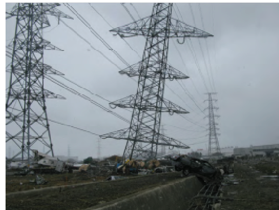
Figure 15. Damaged transmission tower
