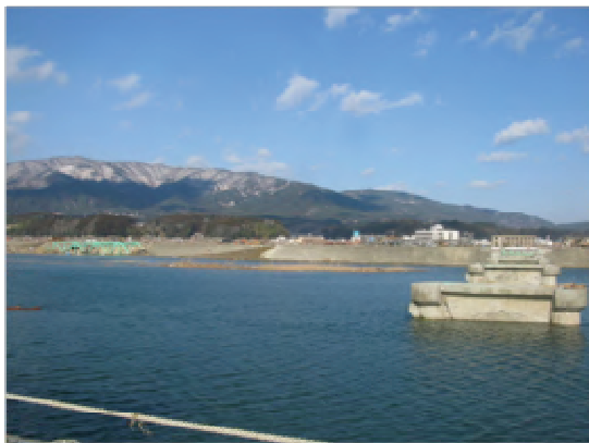
Figure 27. Piers and washed away steel truss
