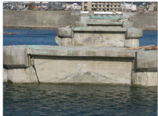
Figure 28. Cracked piers
