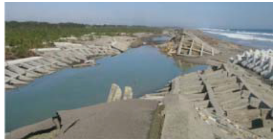
Figure 13. Eroded seawall
