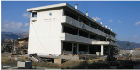
Figure 25. School building foundation erosion
