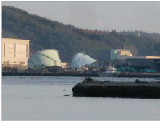
Figure 18. Failed oil tanks
