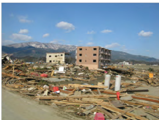
Figure 29. Undamaged newer concrete building
