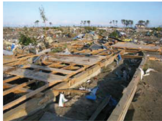
Figure 5. Typical wood frame foundation
