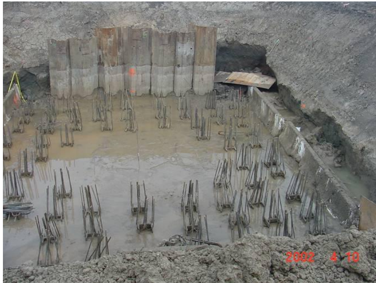
Figure 3.5. Steel (H) piles after driving and re-tapping
