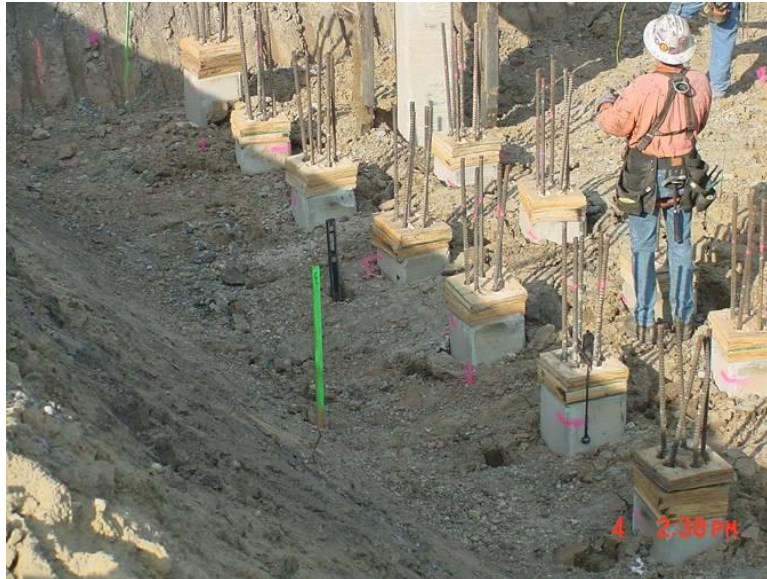
Figure 3.4. Reinforced concrete pile driving
