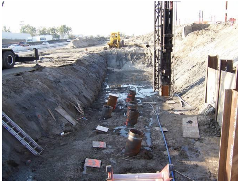
Figure 3.3. Battered steel pipe piles ready for re-tapping)
