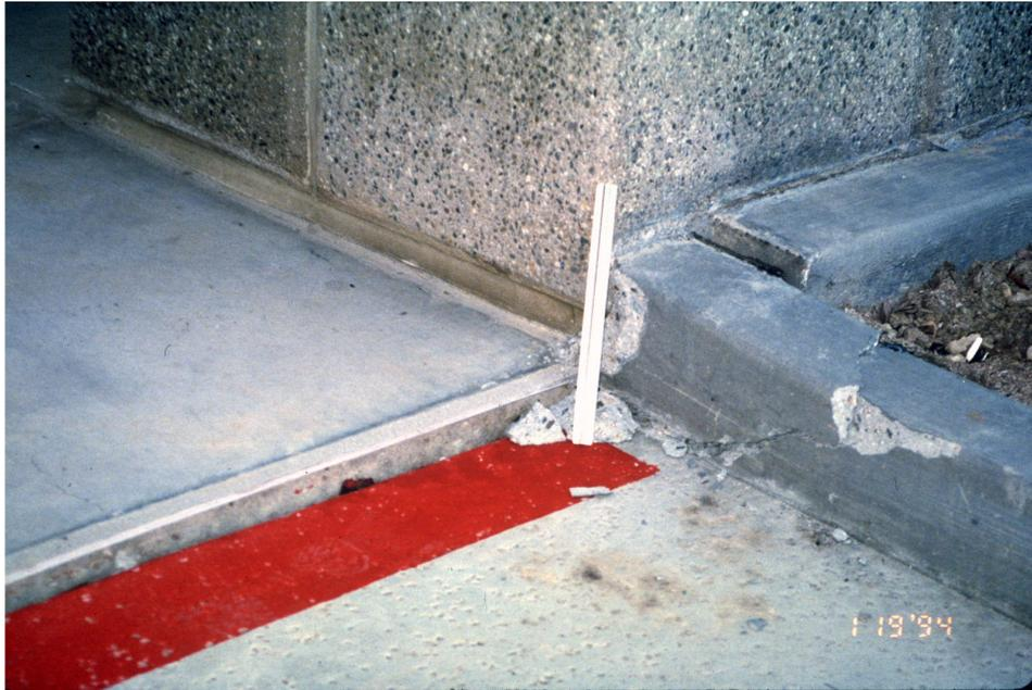
**Figure 2.4.** Liquefaction-induced settlement of exterior slab-on-grade
