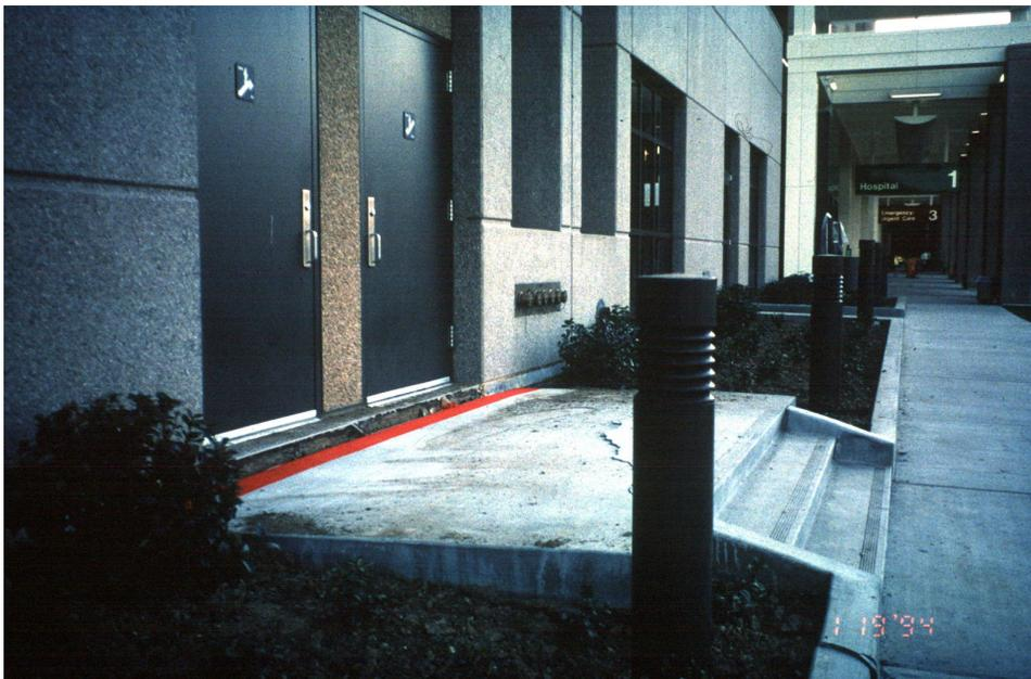
**Figure 2.5.** Liquefaction-induced settlement of exterior concrete steps
