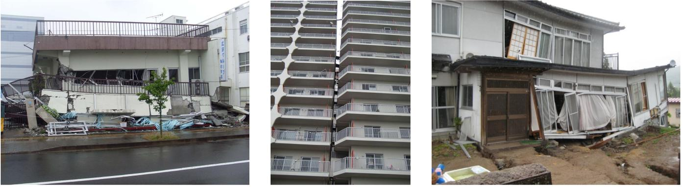
**Figure 5.** Shaking damage in Sendai
