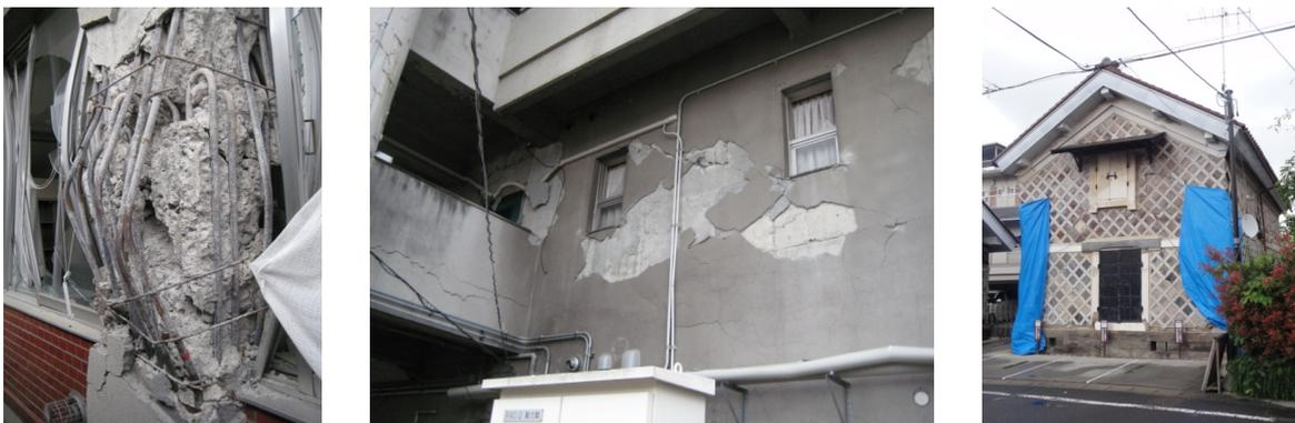
**Figure 7.** Shaking damage in Sukagawa
