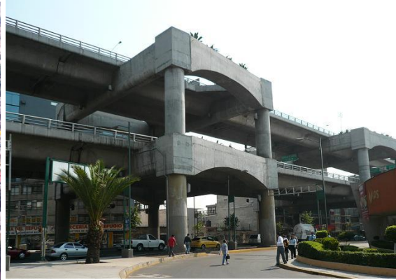
Figure 1.2. Viewing of the double frame structure
