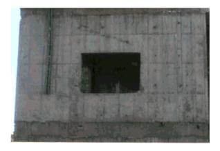
Figure 1: Concrete shear wall with opening (Iran; Semnan 2011)
