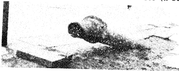
Photo 5. Pushed-out Buried Gas Pipe
