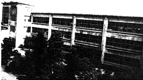
(a) Before Strengthening
