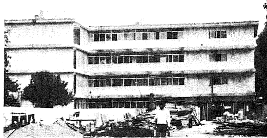
Photo 3 South View of Block E (1986.9)
