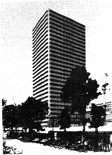
Photo 1 A 30-Story R/C Building
