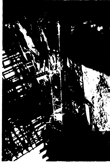
FIG 8 OVERTURNED TOWER CRANE
