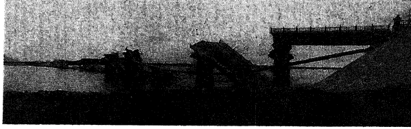
The collapsed Luan River Bridge
