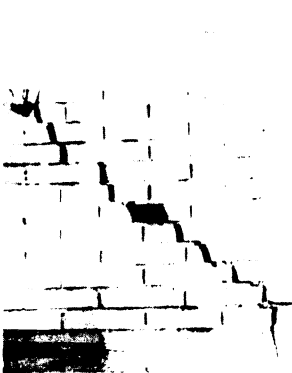
FIG. 7 - Failure along joints for solid brick panels
