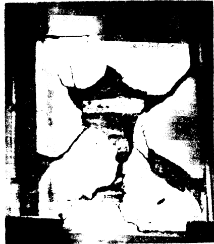
FIG. 2 - Cracks in an actual pier (a); loading scheme (b)
