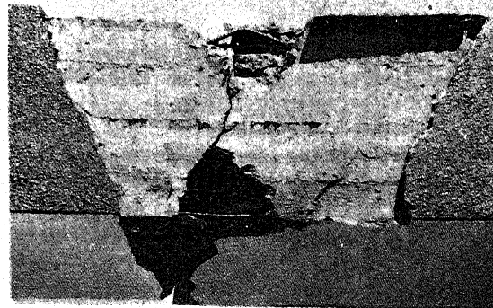
Photo #2. Girder hinge.
