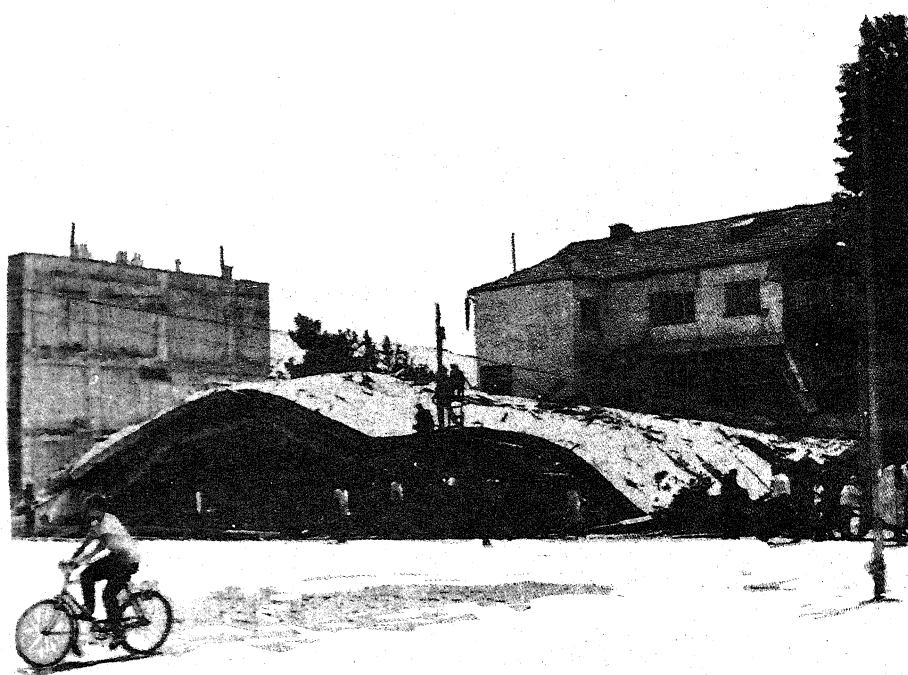
Collapse of the 5 storey S. Bayraklar Building, Adapazarı, Turkey, 1967
