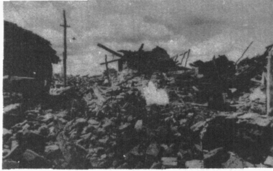
Fig. 2 - Failure of adobe made houses.
