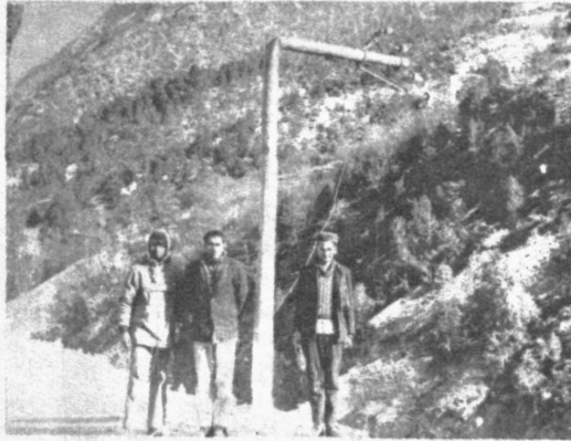
FIG. 1 - TELEGRAPH POLE BENT DUE TO IMPACT OF A FLYING ROCK FRAGMENT
