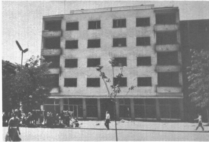
Fig. 1. Soft ground story, Skopje
