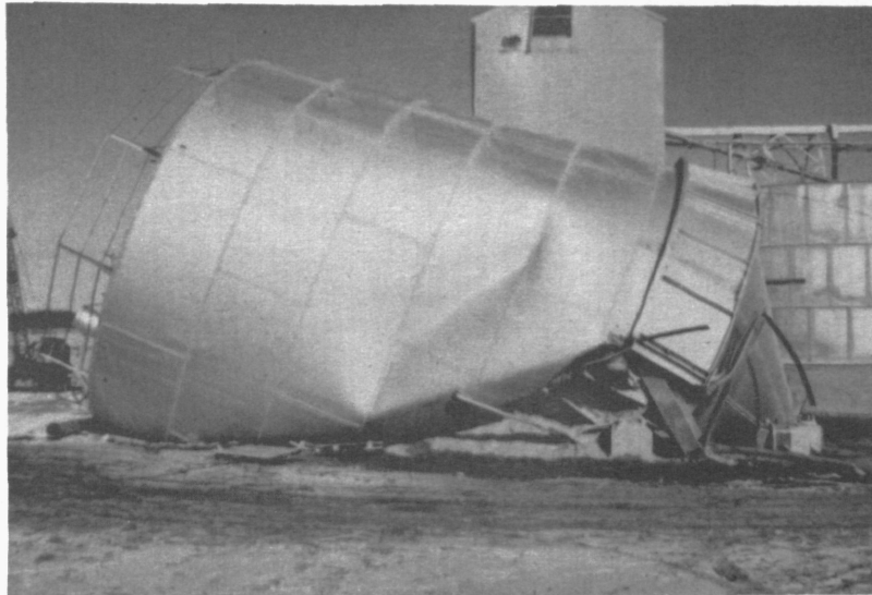
Fig. 5. Collapsed cement bin, Anchorage
