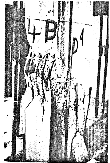
Fig. 7 - Column Failure, Caromay Building
