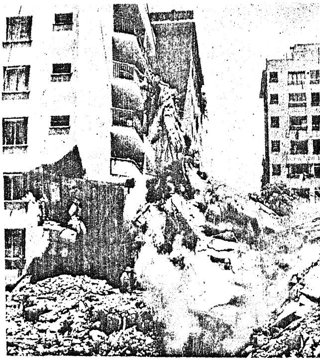
Fig. 23 - Collapse of Mijagual on Nobel Building
