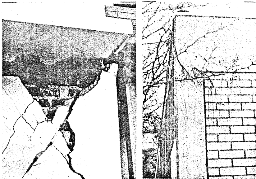
b) Failure of frames confining wall panels
