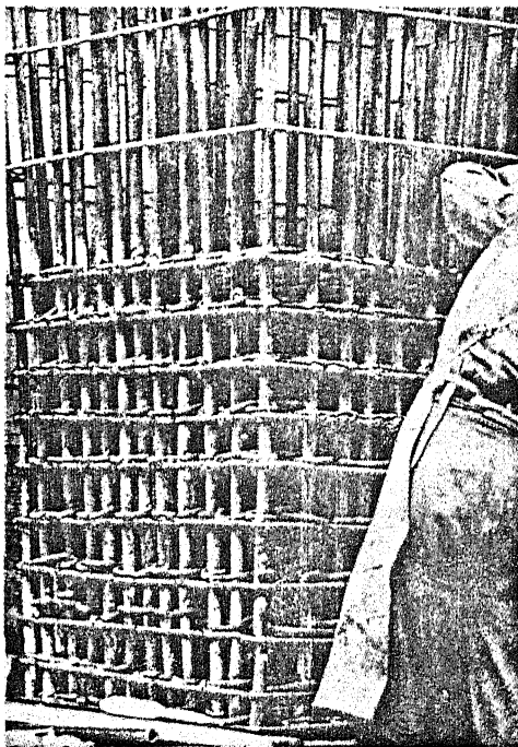
photo 3-Welded grills to increase the ductility of column (see photo 2)
