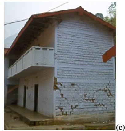
**Figure 5. R/R masonry plastered & decorated to give an impression of dressed stone masonry**
