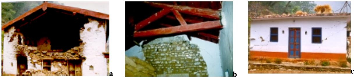
**Figure 6. Failures of R/R masonry walls (a) Gable ends and cross walls (b) Separation of wythes and (c) In-plane shear failure of newly built wall weakened by openings.**
