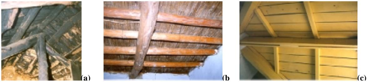
**Figure 8. Typical roof construction (a) Vertical post supporting ridge rafter (b) Framework of wooden logs & twigs and (c) Wooden joist and plank system**
