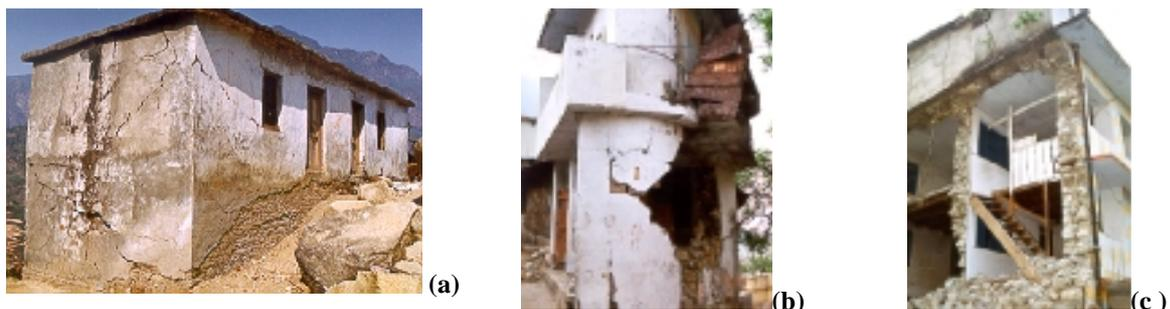
**Figure 14. (a) Vertical irregularity of hill-slope house (b) Non-parallel walls for a corner house and (c) Lack of connection between wall and floor and between exterior and cross walls**
