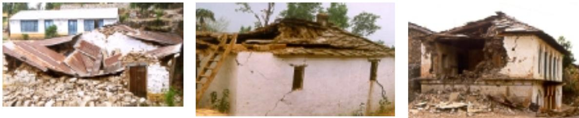
**Figure 9. Collapse of roof structures (a) wall supporting the roof collapsed (b) partial collapse of double pitched roof truss and (c) collapse of wall supporting the roof truss**
