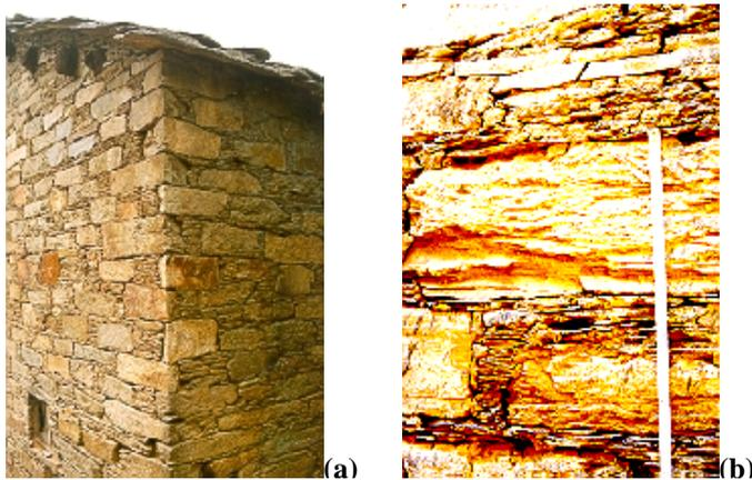
**Figure 4. (a) Traditional stone and slate masonry wall and (b) a close-up view of stone boulder and thin layers of slates**
