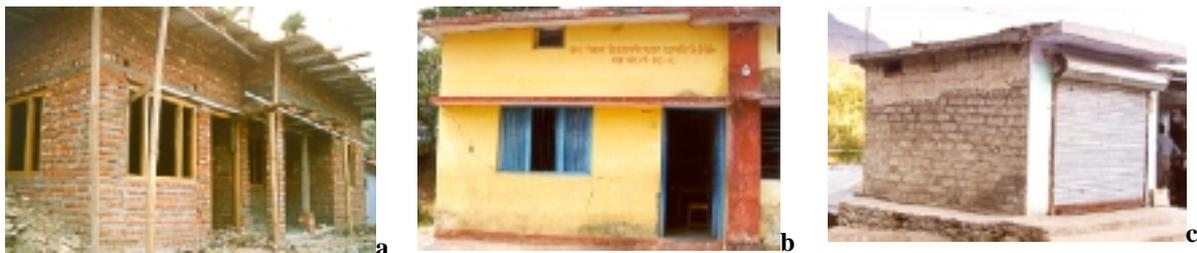
**Figure 7. Brick & block masonry (a) brick house built with lintel bands (b) In-plane shear failure of brick masonry wall and (c) Concrete block masonry construction**
