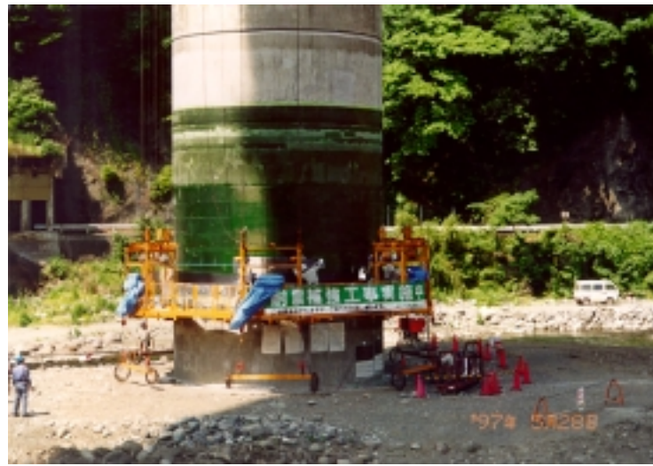
(a) Retrofitted East- and West-Bound Bridge (b) Wrapping of Carbon Fiber Sheets
