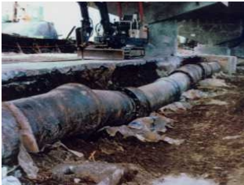
Figure 2: Buried pipelines under earthquakes - ductile iron pipes with seismic joints surviving large permanent ground deformation (left) and brittle failure of cast iron pipes (right)
