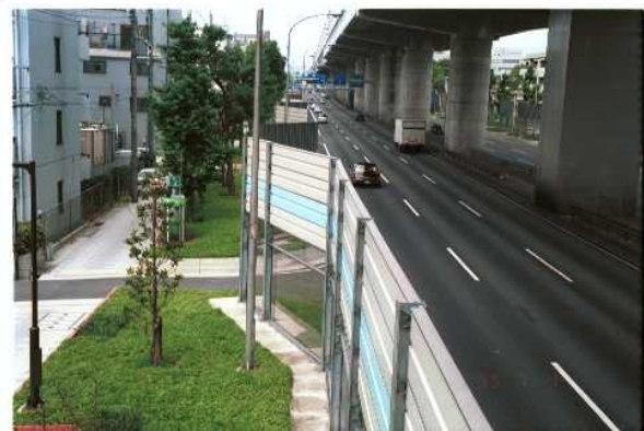
Figure 4: New constructions for improvement of environmental problems from traffic noise adopted in reconstruction from disaster (Ashiya)
