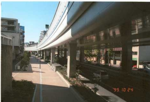
Figure 3: Nineteen-span continuous girder-frame structure with base isolation at pier foot adopted for reconstruction of Benten viaduct in Kobe
