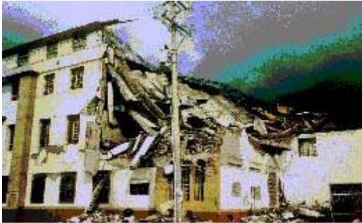
Photo 2: Collaps of unreinforced, non earthquake resistant brick masonry building
