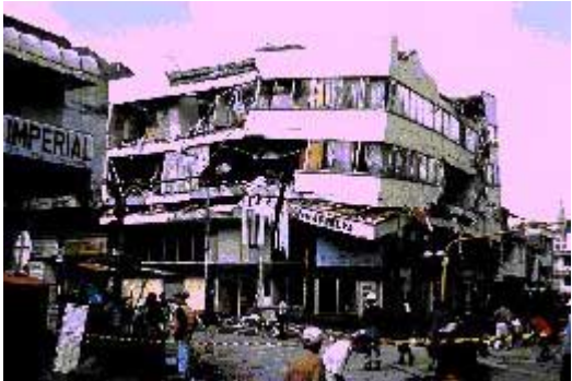
Photo 3: Collapse of old non earthquake resistant building.
