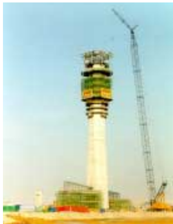
Figure 6. Construction of ATC tower at IIA, Korea
