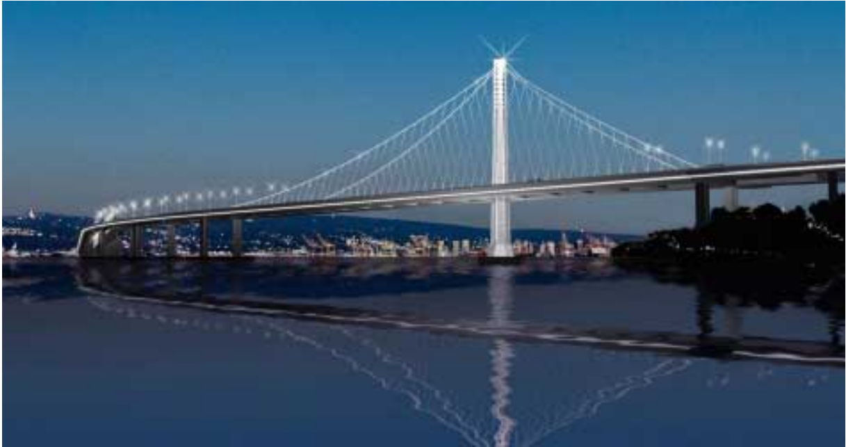
Figure 6. Overview, New SFOBB East Bay Bridge (TY Lin, Moffatt & Nichol, J.V.)
