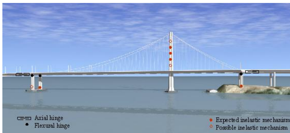
Figure 5. SFOBB East Bay Bridge – Seismic Response Mechanism
