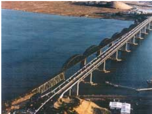
a) Bridge Overview
