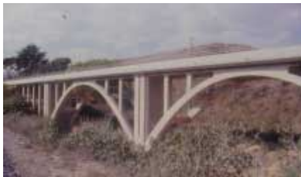
Figure 9 The Arroyo Quemado Bridge After Seismic Retrofit
