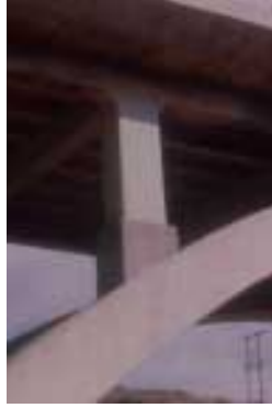
Figure 8 Column Retrofitted Using Reinforced Concrete Jacket And Epoxy Glass Wrap
