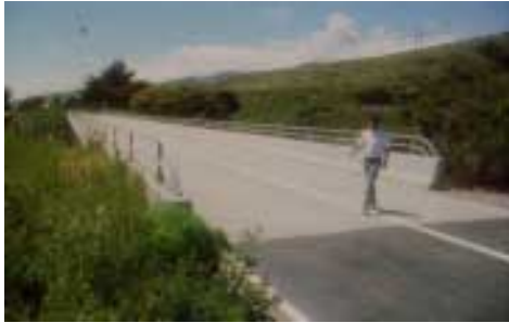
Figure 6 New Reinforced Concrete Deck Overlay
