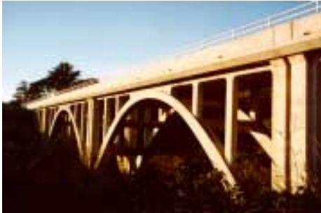
Figure 5 The Arroyo Quemado Bridge Before Seismic Retrofit
