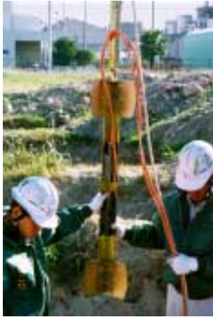
Figure 11: Inclinometer used for investigation
