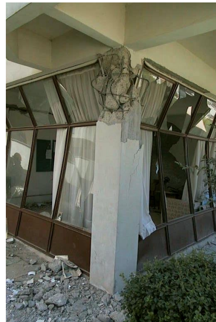
Figure 6. Typical Damage Observed during the 1999 Kocaeli Earthquake in Turkey
