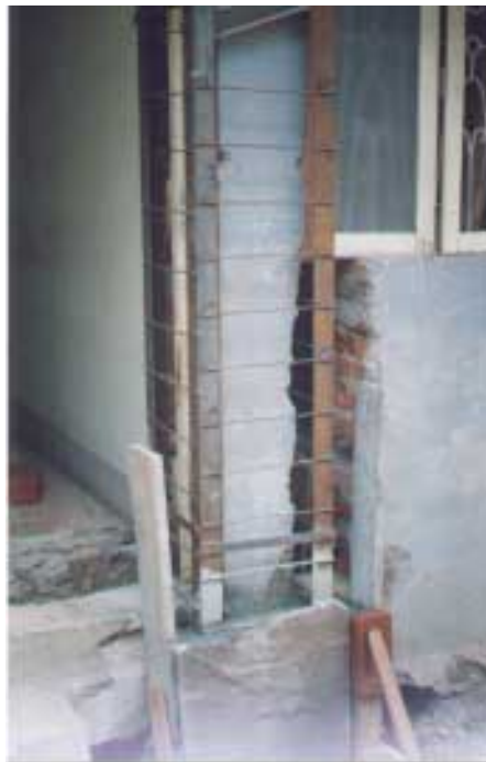
Photograph no.5:-brittle failure of short column supporting staircase midlanding.
