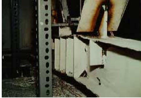
Figure 3. Ductile end-diaphragm specimen having EBF: (a) elevation; (b) hysteretic curves (bolted EBF); (c) shear distortion and local buckling at the link; (d) hysteretic curves (welded EBF)
