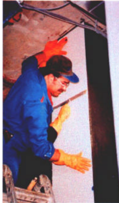
Figure 4 : Port Alberni Federal Building: CFRP Application to Columns with Minimal Disruption
