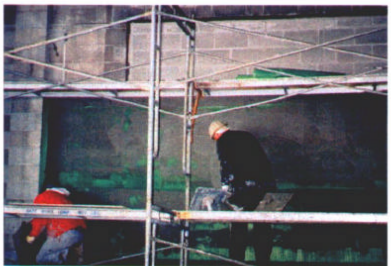
Figure 3 : Standards Building: FRC Application to Masonry Block Walls
