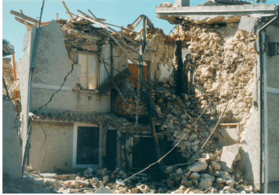
Figure 4. Example of collapse in San Martino village. The building type is characteristic for the whole area. The irregular masonry texture of sample stones is clearly visible. Note the concrete roof in the house on the right. (photo of the author).
