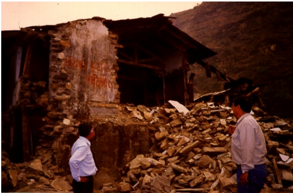
Destruction of rubble masonry and restoration of part skeleton Fig.2
