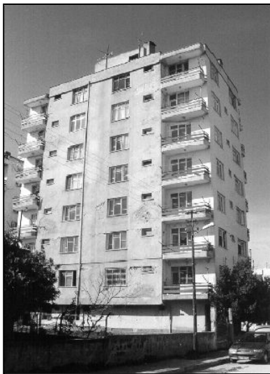
Figure 9. The photo of the 8-story apartment building
