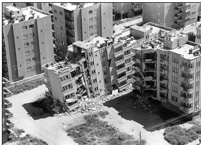
Figure 6. Collapsed and damaged buildings in Ceyhan after 1998 earthquake
