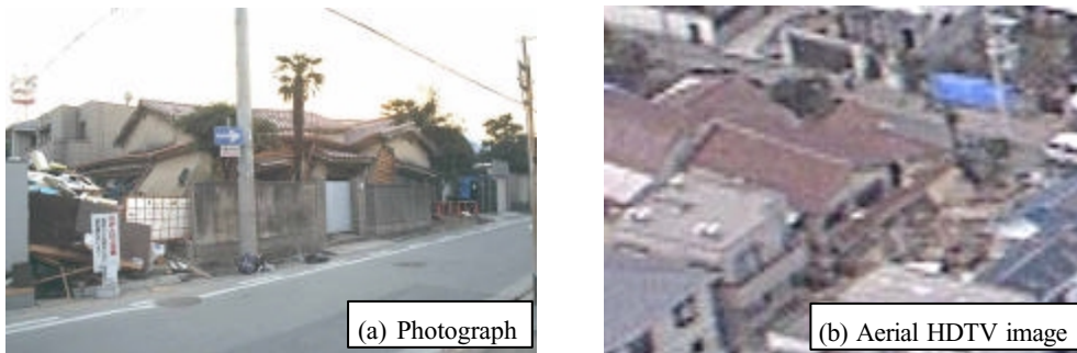
Figure 9: Example of a collapsed building from two different views: (a) a photograph taken from the ground and (b) a snapshot of HDTV images taken from the air
