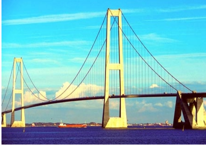
Figure 3 – The Great Belt suspended bridge, in Denmark, passively controlled by flaps
