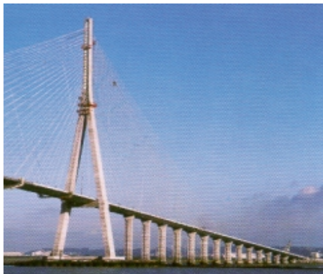
Figure 2 – The Normandie bridge in France, actively controlled during the construction
