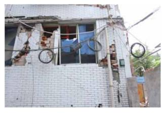
Fig.2 outside longitude wall's damage at the first floor of the traffic administrative bureau
