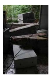
Fig.18 air condition crack by inward collapsed cross wall
