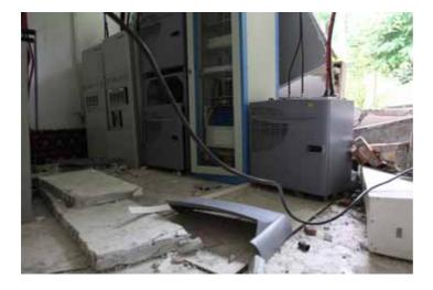
Fig.17 outside cross wall of the communication machine room inward collapse
