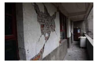
Fig.11 wall damage of first floor at Suiyuan Hotel
