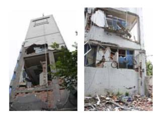
Fig.5 and 6 outside cross wall and cables' damage of three floors of the traffic administrative bureau
