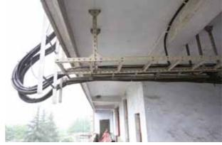
Fig.14 outside cable distribution of communication station
