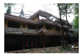
Fig.19 roof collapse of building near the Mount Lingyan cableway
