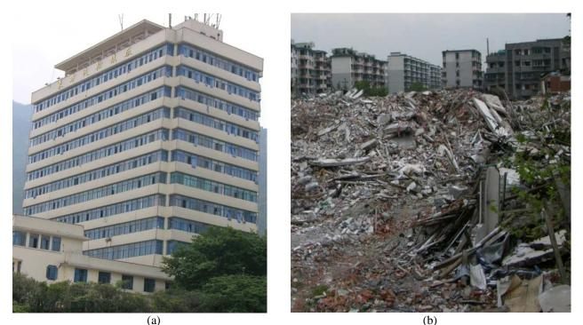
Figure 4: Building damage in the area of the Oriental Turbine factory: (a) an office RC shear wall building with slight to moderate damage, (b) residential CM buildings collapsed (front) and severely damage (rear)
