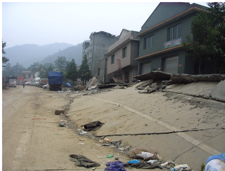
Photo 9 A piece of surface rupture at Renjiaping( 104^{\circ}26'50.3'' , 31^{\circ}48'54.0'' ), which direction turn to Beichuan county, fault scarp is 1.7-2.5m
