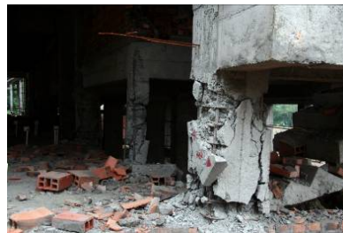
Shear failure of short columns in a split-level RC frames
