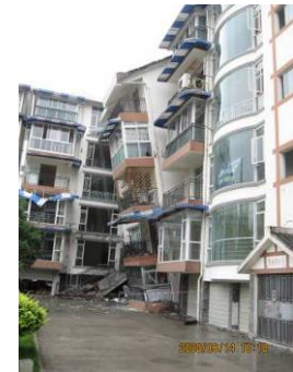
Weak story collapse of a RC frame
