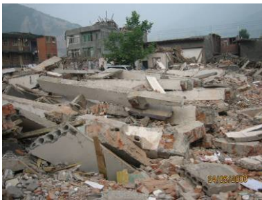
Collapse of the teaching building of Nanba primary school, Nanba
