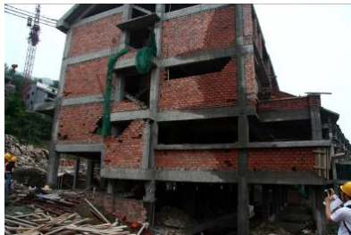
Shear failure of short columns in a split-level RC frames
