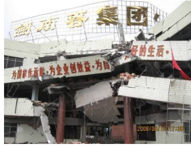
The damage of an office building using horizontal hybrid structure
