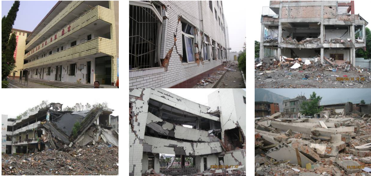
Fig 12 Different states of building damages beyond the design point against severe earthquake
