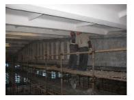
Fig.36 U-shaped steel wire mesh placed on side of the beam
