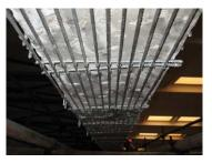
Fig.35 Steel wire mesh placed on bottom of the beam
