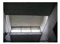
Fig. 10 Protrusion of the skylight of the plant building cracked horizontally
