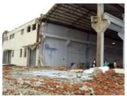
Fig. 11 Bent gable of the plant building completely collapsed
