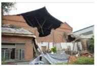
Fig. 7 Gable masonry of plant buildings without ring-beams almost completely collapsed
