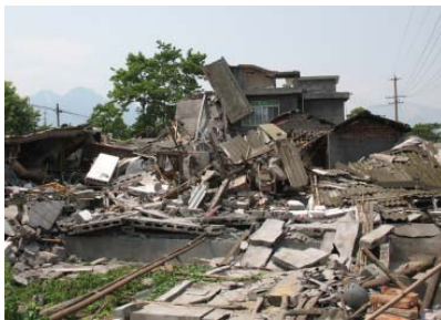
Figure 23. Collapsed residential units
