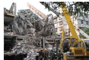
Figure 22. Collapsed Bank of China branch
