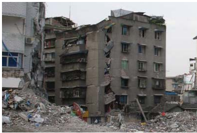
Figure 12. Collapsed wing
