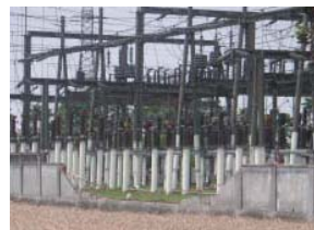
Figure 28. Collapsed URM wall at a substation
