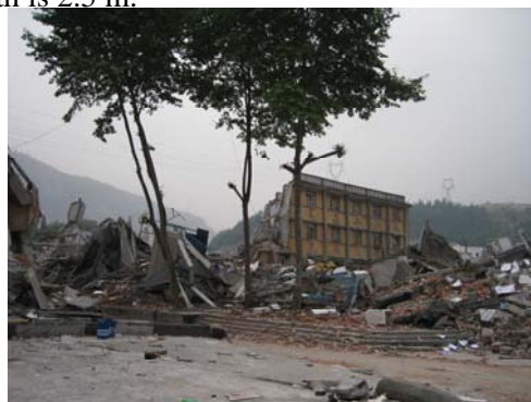
Fig13. the office building of the power station
