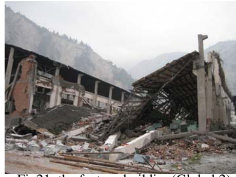
Fig21. the factory building(Global 2)
