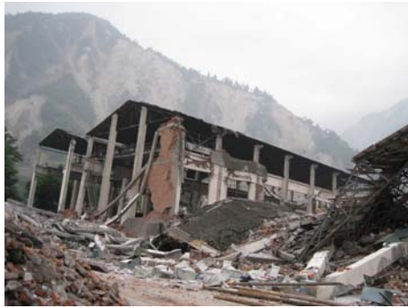
Fig20. the factory building (Global 1)
