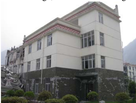
Fig2. the office building of the Yingxiu secondary school(Local 1)
