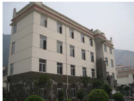
Fig3. the office building of the Yingxiu secondary school(Local 2)
