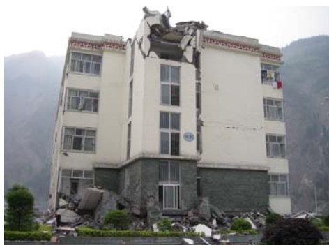
Fig10. the student dormitory of the Yingxiu secondary school
