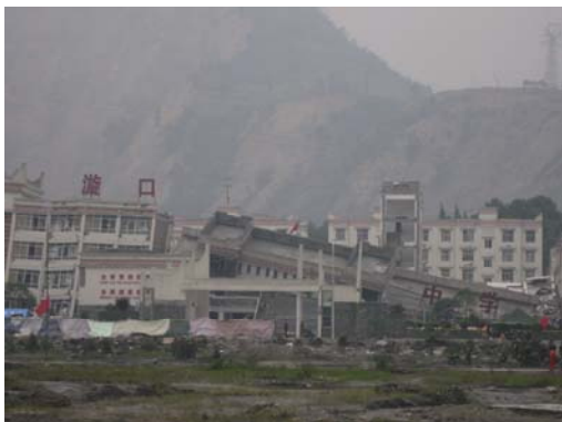
Fig5. the complex building of the Yingxiu secondary school (Global 1)
