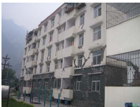
Fig12. the teachers residential building of the Yingxiu secondary school
