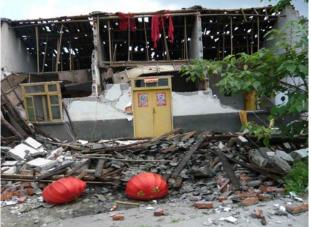
Fig. 14 Collapse of the front wall of a rural house in Zundao town, May 14, 2008
