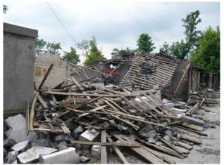
Fig. 16 Collapse of walls and wood roof of a rural house in Guangji town, May 14, 2008
