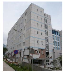
Fig. 3 Shear crack of the bottom two stories of an office building in Dongfang Steam Turbine Works, Hanwang town, May 15, 2008
