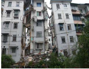
Fig. 5, A special destroyed building near the secondary surface rupture in Hanwang town, May 15, 2008
