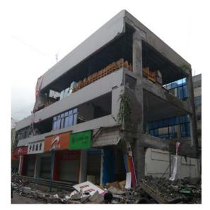
Fig. 4 Collapse of the exterior walls of a three-story cast-in-situ RC frame structure in Hanwang town, May 15, 2008
