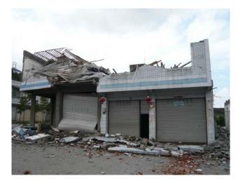
Fig. 11 Collapse of the top floor of a bottom-frame building in Zundao town, May 14, 2008
