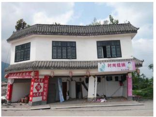
Fig. 12 Inclination of columns of an imitation of ancient building in Jiulong town, May 14, 2008
