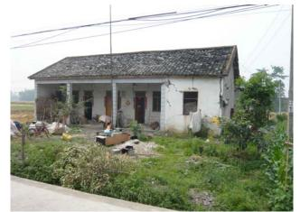
Fig. 13 A moderate destroyed rural house with severe cracked walls, Mianyuan town, May 16, 2008
